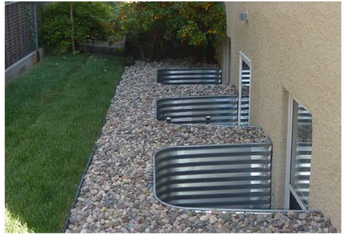
After: The decision was made, says Orfield-Skrivseth, to fill the space previously filled with concrete with sod, rocks and egress windows. The galvanized window wells were chosen because they are cost-effective and are easy to keep clean.
