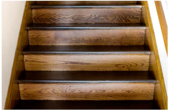
After: Once the linoleum was peeled off these existing wood stairs, all that was required was a sanding and staining, Orfield-Skrivseth says. A very cost-effective project that only takes three to four days altogether, but completely changes whether you want to walk on the stairs or not, she says.
