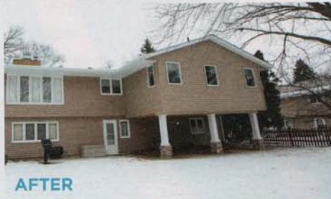
Before and after photos of the cantilevered addition that provided the Roberts family space for a new 415-square-foot master suite.
