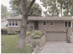
1425 Flag Avenue South Tuck Under Garage Multi Room Renovation
