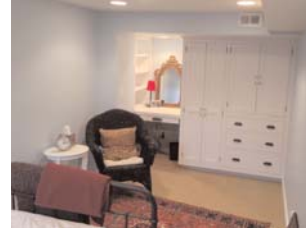
3809 Glenhurst Avenue South Colonial Basement Renovation
