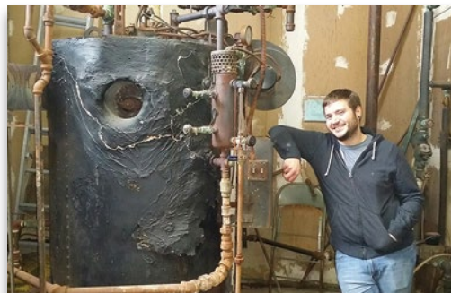
BEFORE: James Turitto with their 30-year-old Fulton Boiler.
