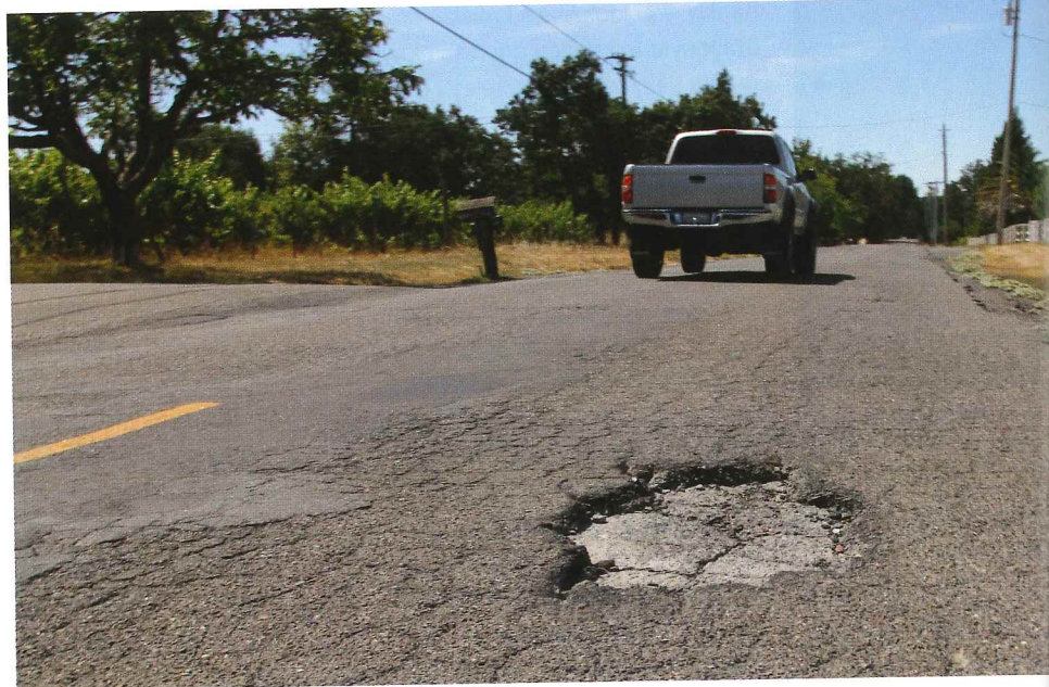
Santa Rosa's heavily traveled Willowside Road is known for its many potholes. [Duncan Garrett Photography]
