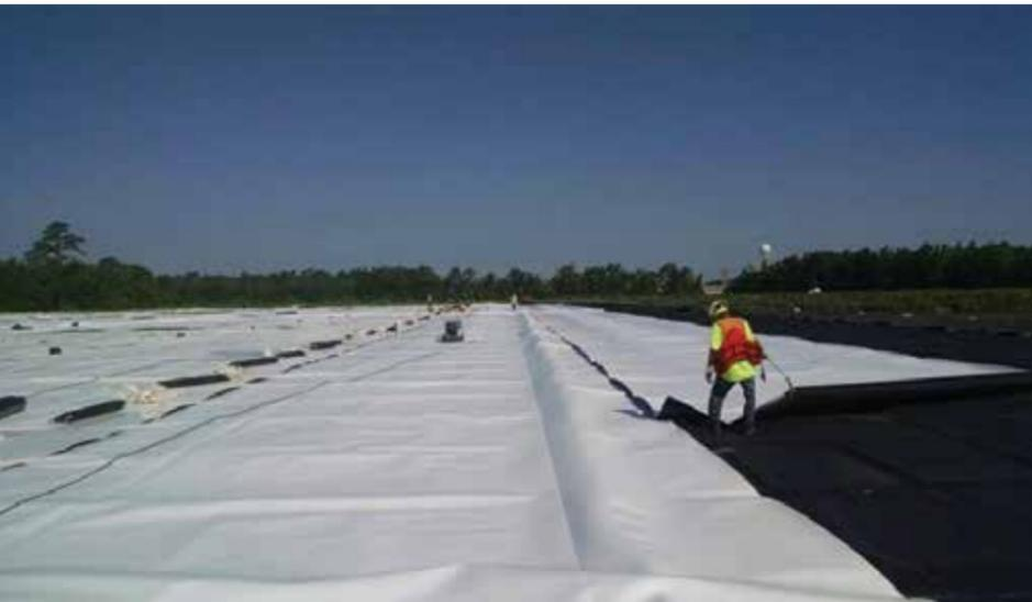
PHOTO 2 The geogrid was installed to distribute surface loads across a wider area.
