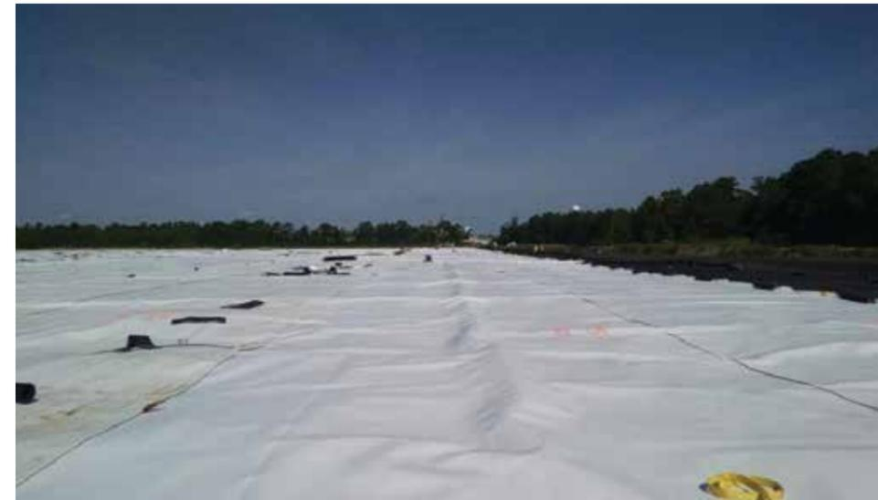
PHOTO 3 A white 80-mil HDPE geomembrane was installed, stretching across the entire 12-acre basin.
