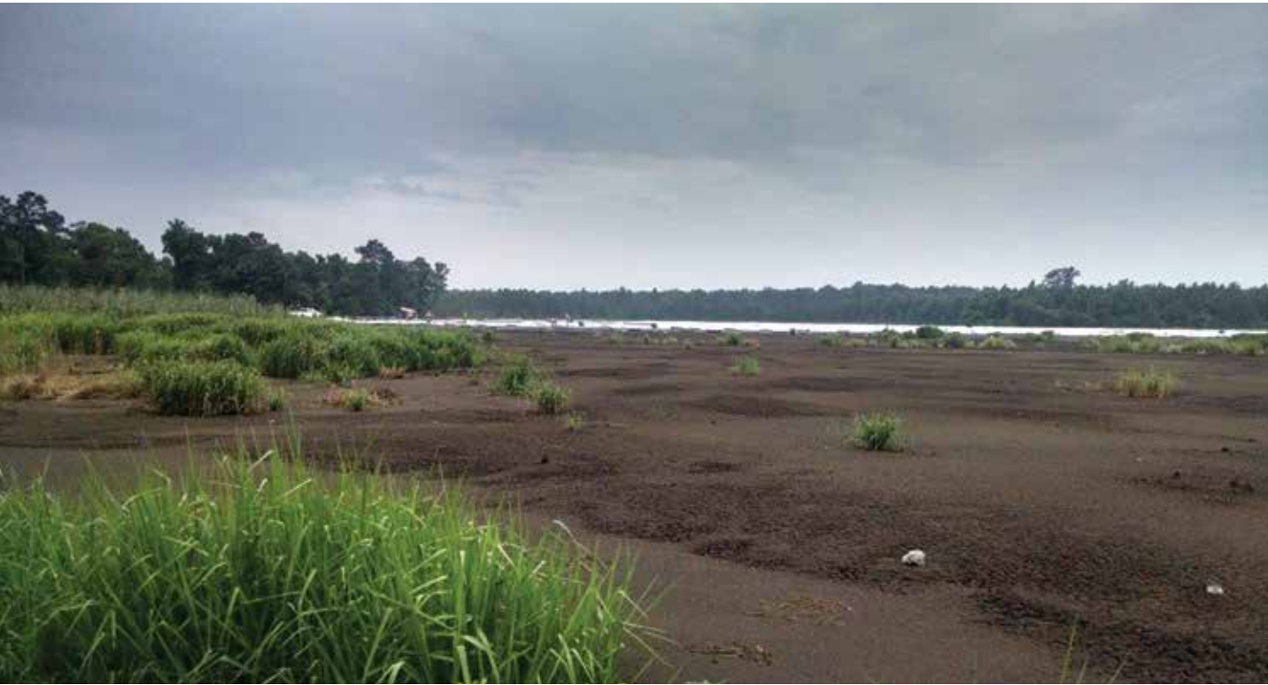
PHOTO 4 The geomembrane was buried in a perimeter anchor trench and backfilled.
