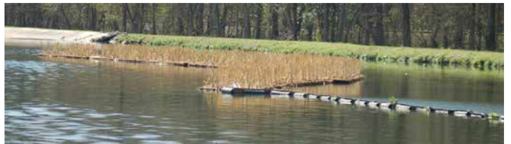
The brown grasses of the BioHaven Floating Treatment Wetlands in the Maringouin sewer pond are shown in the photos above.
