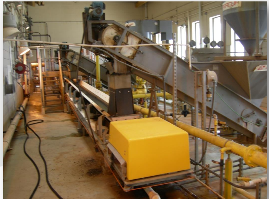
GRIT BELT CONVEYOR
