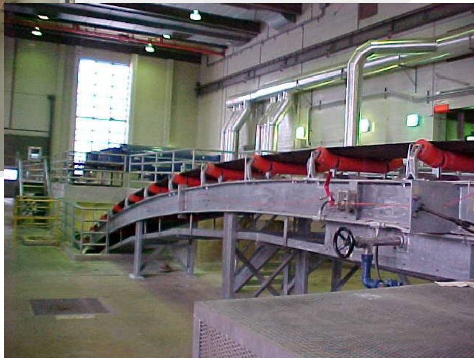
VERTICAL CURVE BELT FILTER PRESS SLUDGE St. Paul, Minnesota
