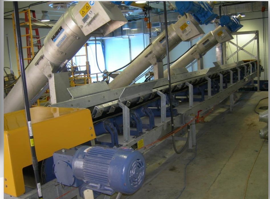
FINE SCREENINGS Sioux Falls, South Dakota Fiberglass drive end guard
