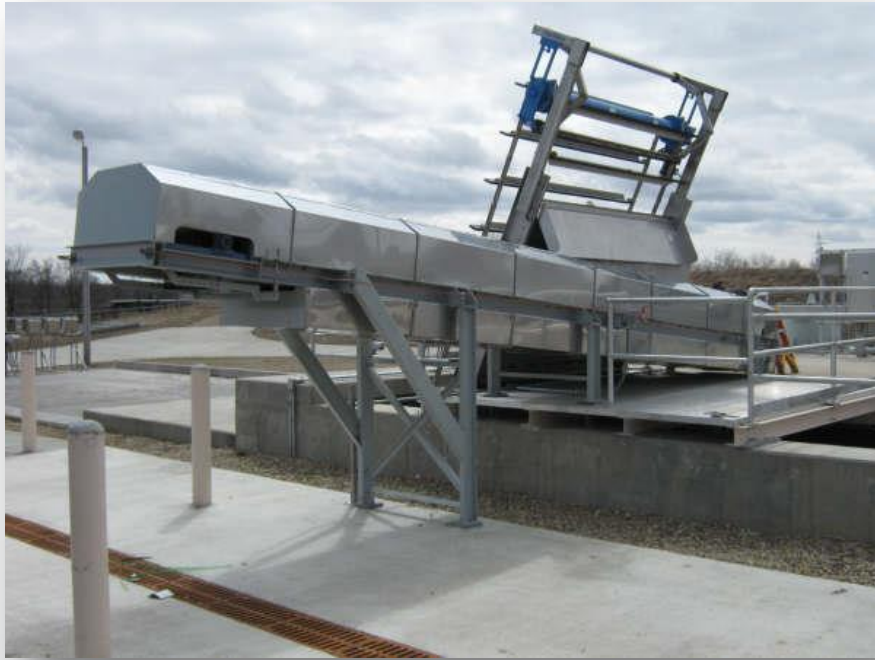
SCREENINGS BELT Bloomington, Illinois Completely Enclosed & Insulated
