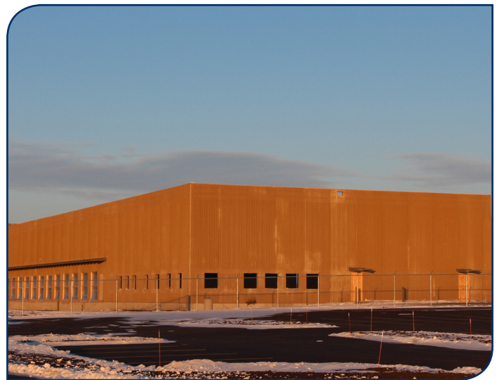
New Fed Ex building under construction in Mankato.
